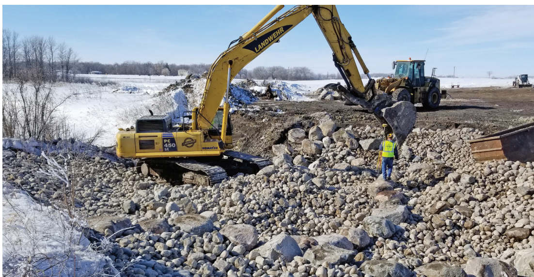
Almost finished! The new rock arch rapids will keep the Sand Hill Lake level high, while also making it easier for migrating fish to cross into the lake.
